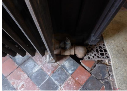
St Mary's heating has not worked for years, the floor, covered by the Victorians in impermeable tiles, has suffered from damp. Work is urgently needed to install new heating, electrics, boilers, kitchen facilities and floor.
