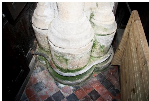
St Mary's heating has not worked for years, the floor, covered by the Victorians in impermeable tiles, has suffered from damp. Work is urgently needed to install new heating, electrics, boilers, kitchen facilities and floor.
